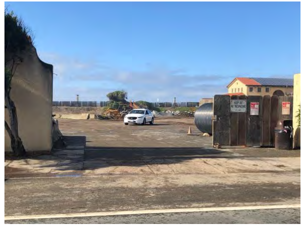
The Sharp Park Pump Station is undergoing an odor control upgrade to make it compatible with any future redevelopment of the 2212 Beach Boulevard site.
