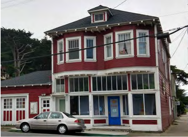
Anderson's Store (220 Paloma Avenue). Built in 1907, Anderson's Store was the first general store and telephone switchboard for the area, the control point for the eater supply for the neighborhood, and the first source of gasoline for automobiles using a hand-crank pump.
