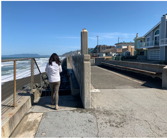
Direct beach access is provided at San Jose Avenue.
