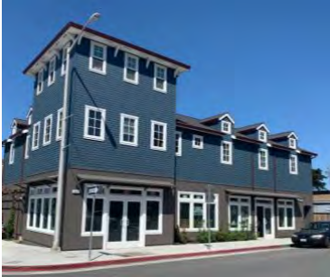
1. This contemporary building at 1680 Francisco Blvd. mimics the style of the Little Brown Church. Retail and residential parking is behind the building.
