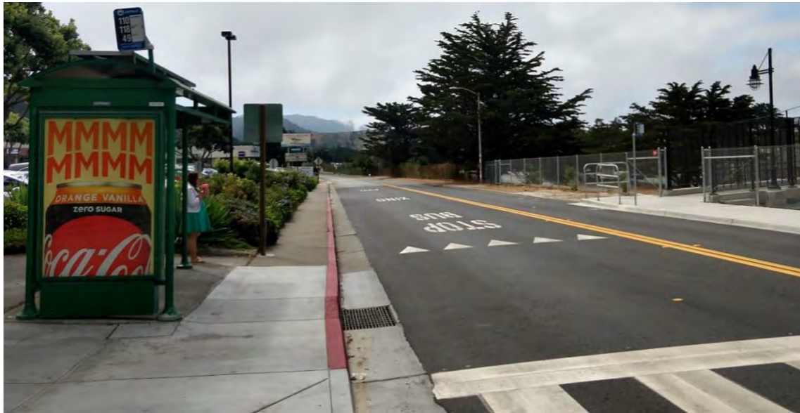
View looking south down Oceana Boulevard along Eureka Square Shopping Center. Street improvements such as the new overpass, crosswalk, signs, plantings, and bus shelter help improve the pedestrian experience.
