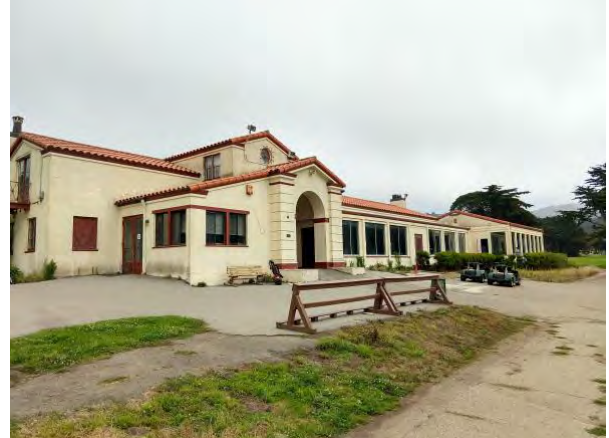
Sharp Park Golf Course and Clubhouse (2600 Francisco Boulevard). Located to the south just outside of the Planning Area, the Golf Course dates to 1929 and was designed by famed golf course architect Alister MacKanzie in the classic "Links" style near the ocean and sand dunes. The Clubhouse, built in 1932, includes a bar, restaurant, and golf shop.
