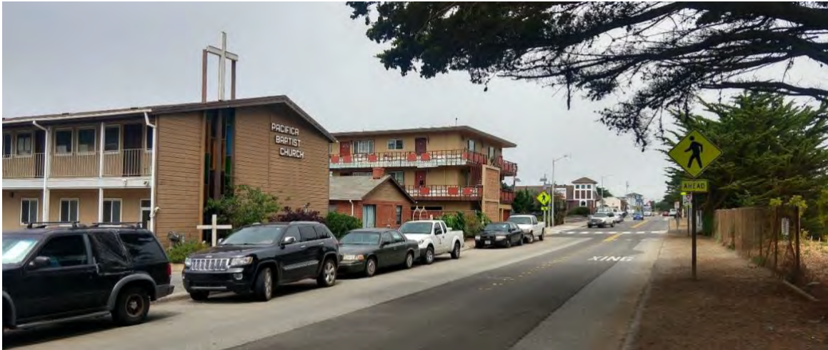
View looking northbound along Francisco Boulevard. This picture shows street crossings for the new pedestrian overpass as well as the Little Brown Church in the distance.
