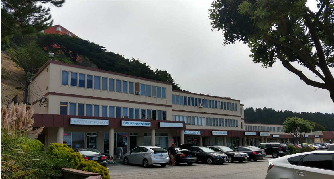
The Eureka Shopping Center is located to the East of Highway 1 in the Sharp Park Specific Plan area.
