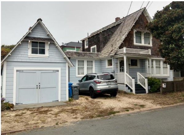
Private residence (185 Carmel Avenue). Designated as a Historic Landmark in 1985, this home appears to be built in coastal cottage style with a pitched gable roof, wooden shingles and wood lap siding.
