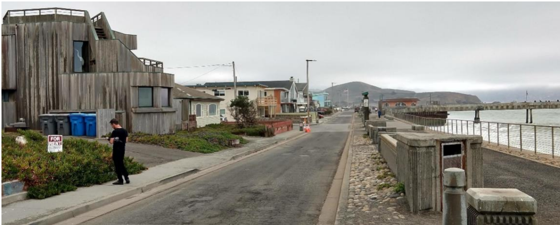
View of Beach Boulevard looking south. Residential properties are located on the left side and the beach promenade is visible on the right. The Pacifica Municipal Pier can be seen in the distance.
