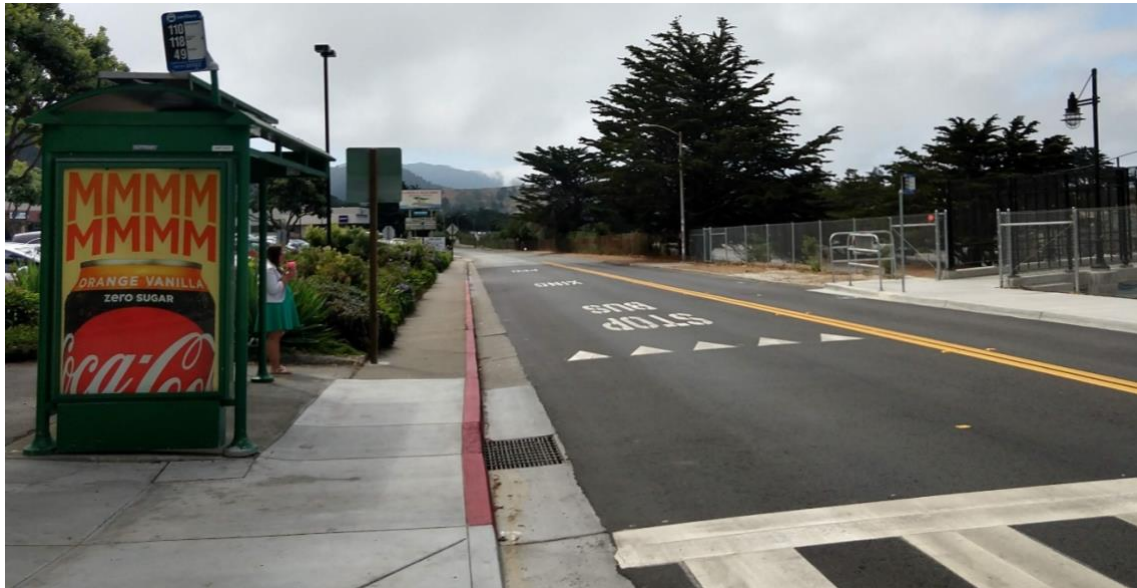
View looking south down Oceana Boulevard along Eureka Square Shopping Center. Street improvements such as the new overpass, crosswalk, signs, plantings, and bus shelter help improve the pedestrian experience.
